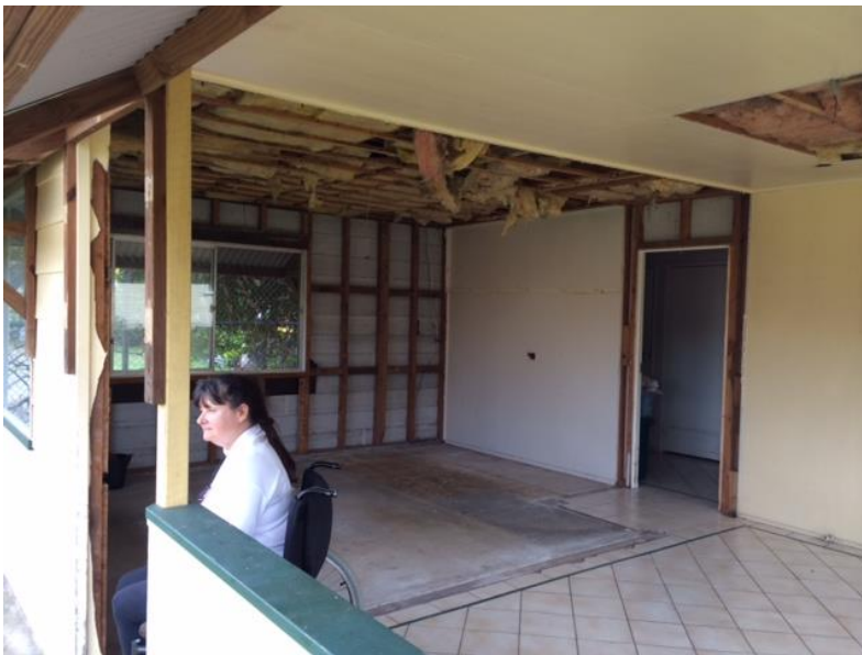
My bedroom & patio demolished.
